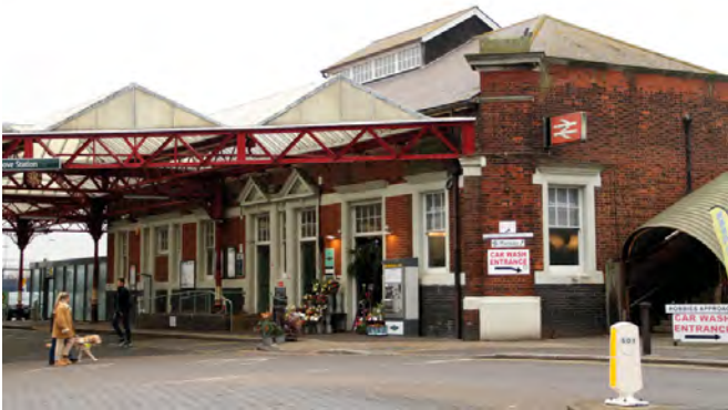
Figure 3.7: Hove Railway Station and footbridge
